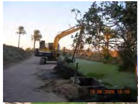
Figure 19: Mechanical removal of aquatic vegetation from Hammad Canal, El Burullus area (CU10)
